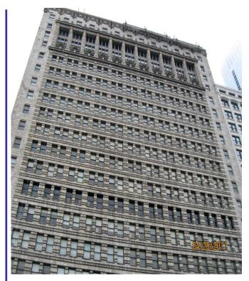
Mueller & Associates, LLC (MA) provided critical inspection services to the building in 2009 and designed and oversaw construction of a complete terra cotta cornice restoration 2010. Building is Illinois & Chicago Landmark. Because the Cornice is landmark, extensive expertise of terra cotta elements was required by the property.
